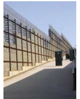
above left to right: Interior of the Apartheid Museum; Rear façade of Arts Center at the University of Johannesburg; Entry ramp to the Apartheid Museum with wall of loose stones in the metal "cages". All courtesy of Mashabane Rose Associates.
