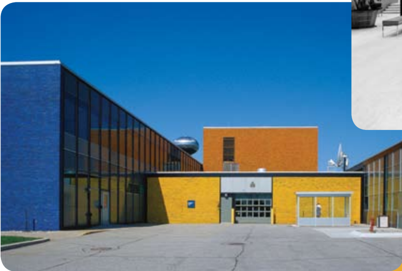
above: View of General Motors Technical Center showing color glazed brick. © Balthazar Korab Ltd.
